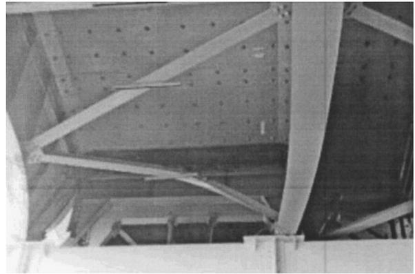
**Fig. 4.** Damage to end cross frames and girders during 1995 Kobe earthquake
