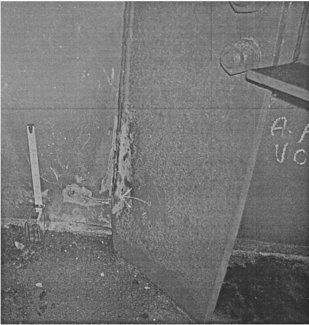
**Fig. 3.** Damage to web stiffeners during the 1994 Northridge earthquake (Astaneh-Asl et al. 1994)
