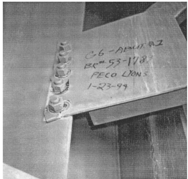
**Fig. 2.** Damage to end cross frames during the 1994 Northridge earthquake (Astaneh-Asl et al. 1994)
