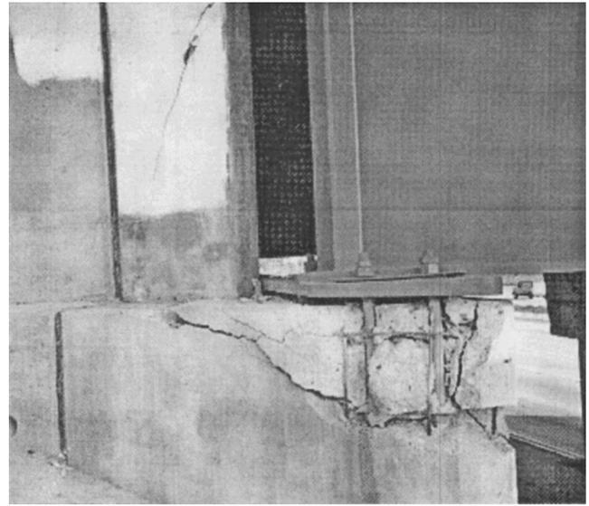
**Fig. 1.** Damage to bearing during the 1994 Northridge earthquake (Astaneh-Asl et al. 1994)
